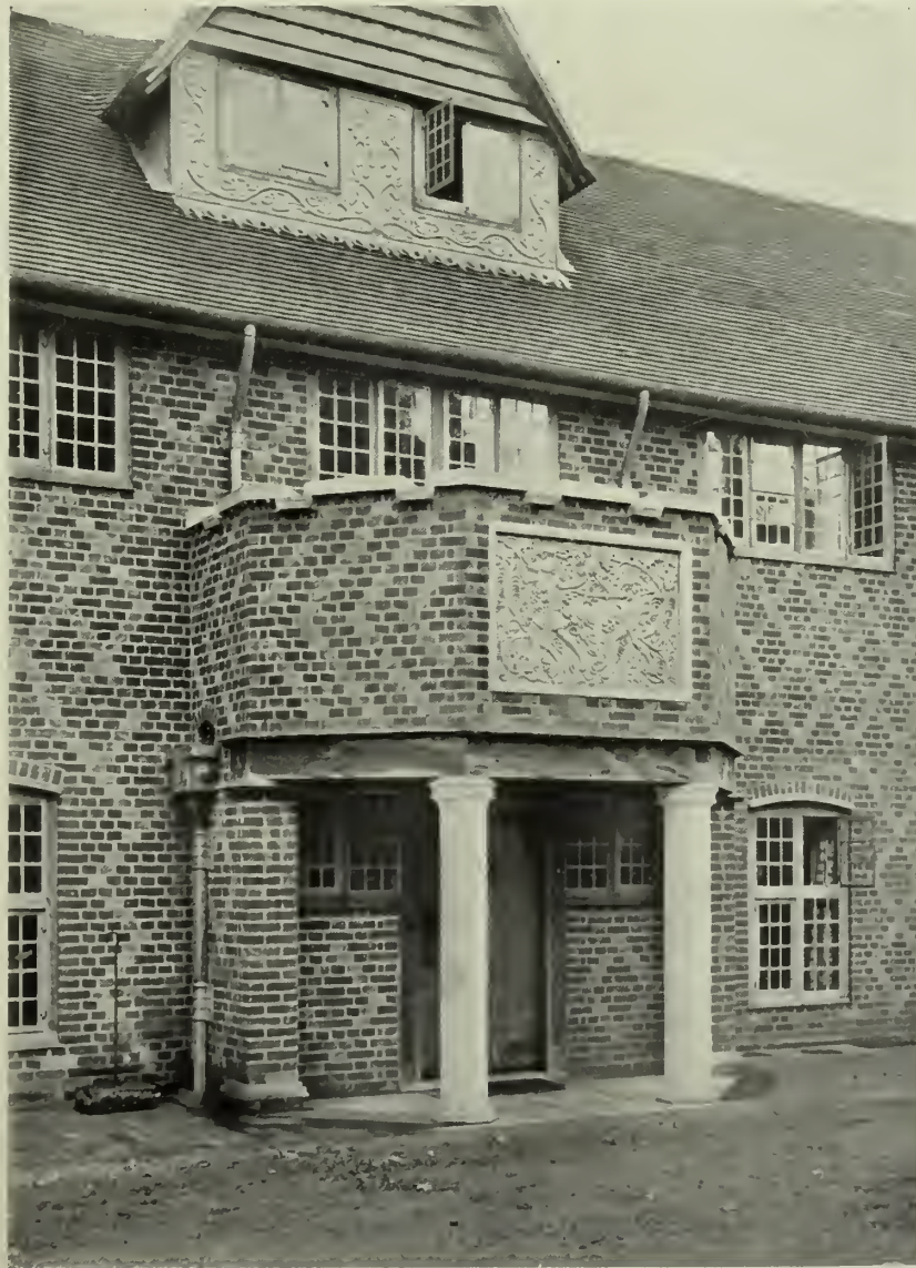
NORTH ENTRANCE TO "SANDHOUSE," WITLEY, SURREY.
